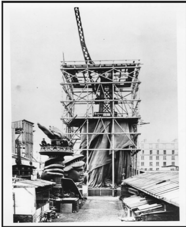
Statue of Liberty under construction in Paris, 1886
